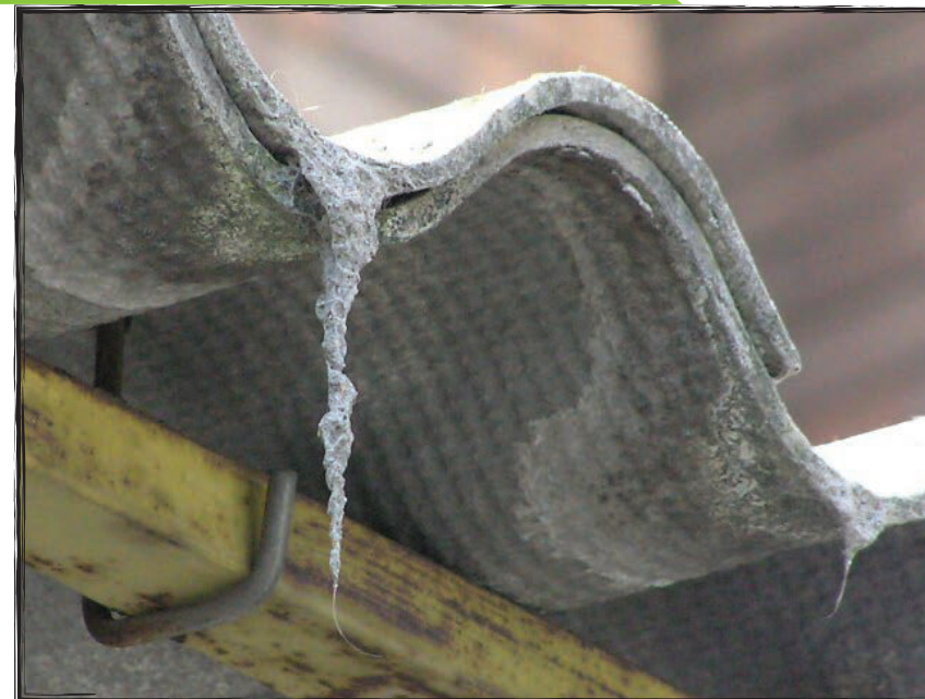
CHAPAS DE FIBROCEMENTO (ASBESTO-CEMENTO)
